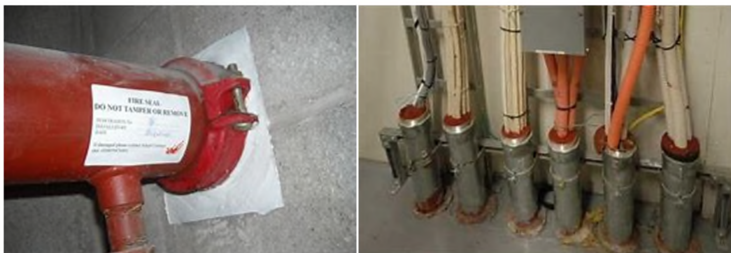
Figure 4: Fire Stopping Through Walls and Floors
